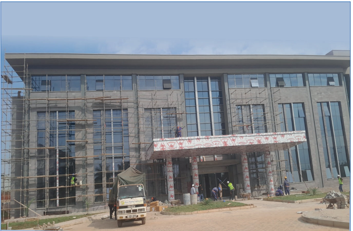
(Below) the same under construction
